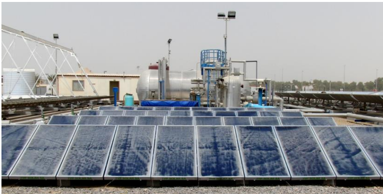
Dust accumulation increases sunlight scattering (diffuse)
